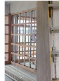
Steel Frame + Studs Base Board Not Required
