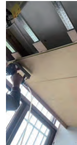
Directly On Steel Frame
